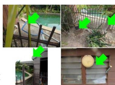
A minimum 300 mm clear NCZ must be maintained to the internal barrier.
